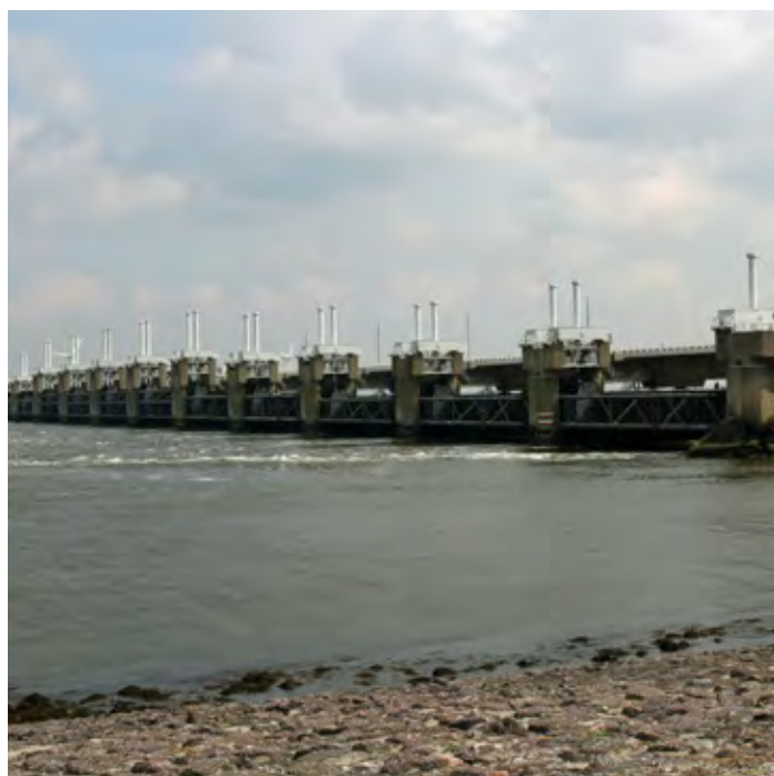
The Oosterschelde flood barrier is the largest and most famous of the Delta works. The 9 km-long storm surge barrier seals off the inland sea Oosterschelde from the North Sea when there is a threat of high water. The barrier has been in use since 1986.
